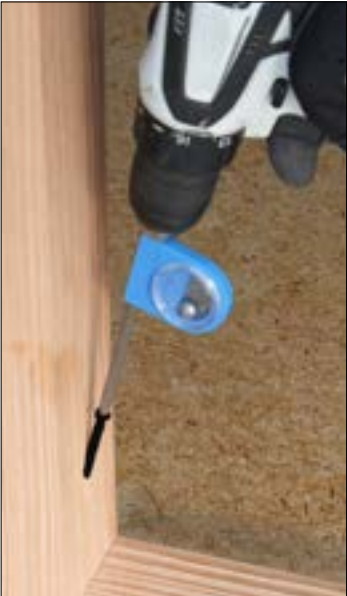
Typical WSTS45-EXT stud to bottom plate installation
