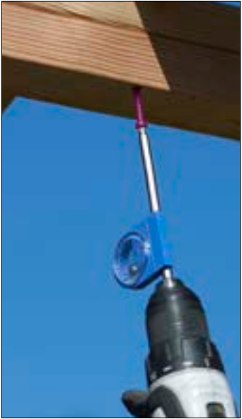
Typical WSTS6-EXT truss to top plate installation
